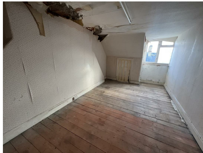
Access to under eaves storage, exposed wooden floor, window to fore.
