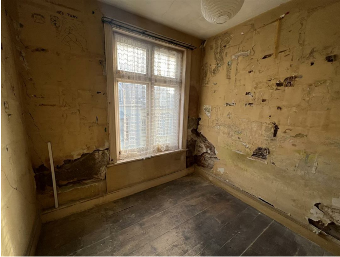
Window to fore, exposed wooden floor.
