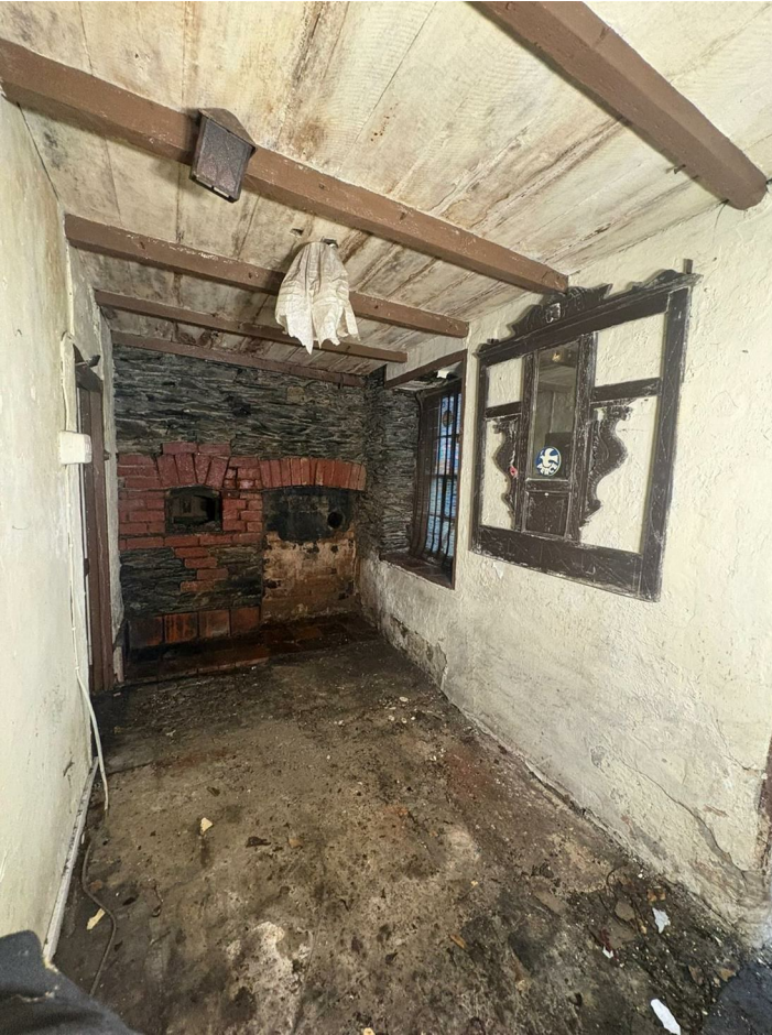
with an old bread oven, window and door to rear. Door to
