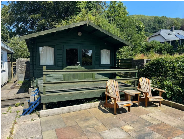
Currently utilised as an office. Inclusive of sauna.
