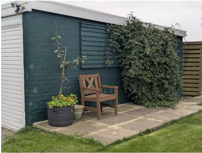
with up and over door and power connected.
