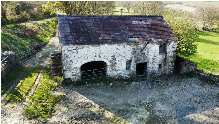
stables with loft over
